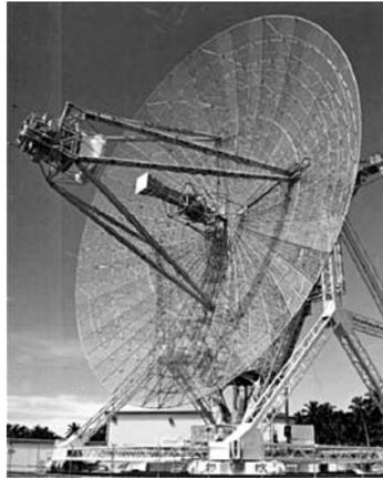
Figure 5: Multipurpose RADAR Antenna
